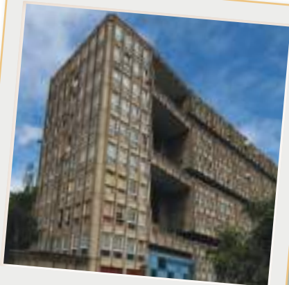
Robin Hood Gardens Estate in Poplar
